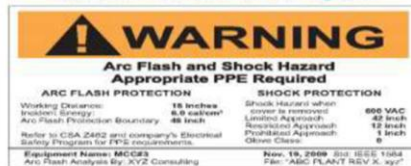
Example of Detailed Arc Flash and Shock Warning Label
