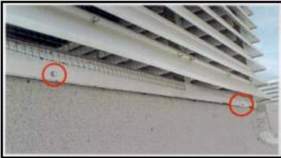
Inadequate securement
