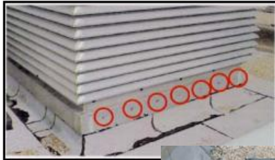
Adequate securement
