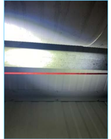
Linear Heat Detection Cable (155 F)
