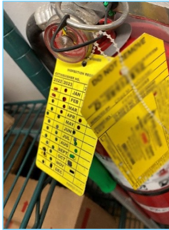
Monthly Fire Extinguisher Checks and Annual Inspection Tag
